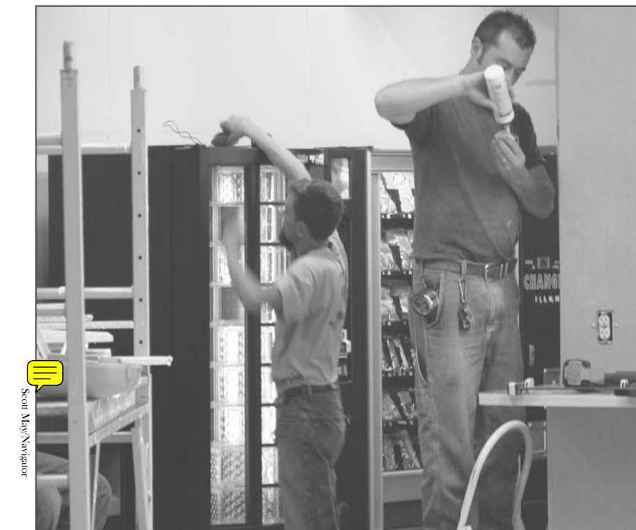
Vending machines are being put in to occupy the space left vacant by Common Grounds building.
